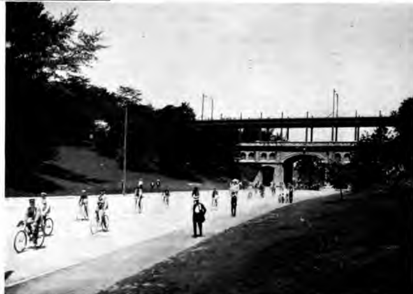
EDEN PARK, CINCINNATI. The Main Entrance, Gilbert Avenue.
